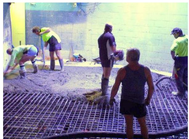
Laying new concrete on the new, stronger, foundations.
